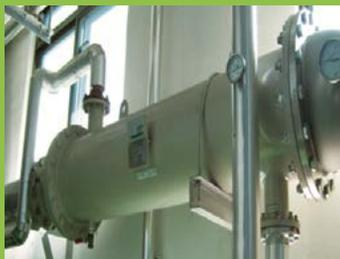
Recycling coolant of air compressor
